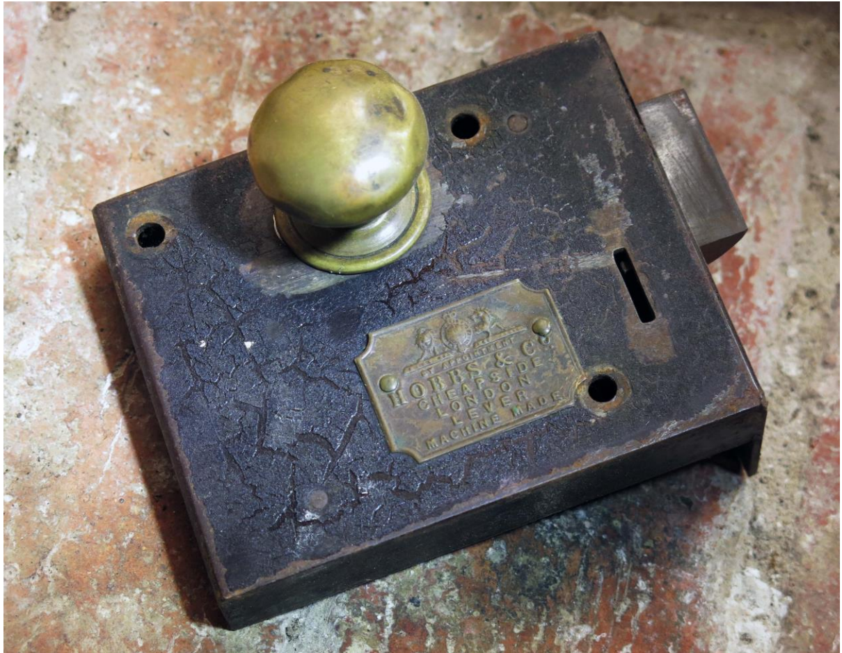
Hobbs & Co lever rim lock in storage at 'Mintaro' Moneggeetta, Victoria: Miles Lewis.
