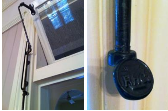
US patent 626213 to W T Adams, 6 June 1899, for a transom lifter. Transom lifters in a house at Auchenflower; the locking mechanism bearing the patent date, and the handle bearing the brfnd of the Reading Hardware Company. Illustrations provided by Magnus Eriksson.
